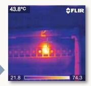
The thermal image clearly shows a defect or an overheated fuse. It can have very severe consequences. An entire production line can be shut down for several hours if this problem is not timely fixed.
