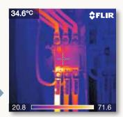
Loose or badly connected cables start to overheat. If left unrepaired, heat can rise to a point where cables start to melt or, even worse, set the environment on fire.
