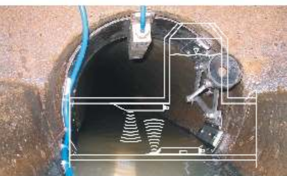
Air-ultrasonic, water-ultrasonic and hydrostatic measurement - investigation of channel efficiency
